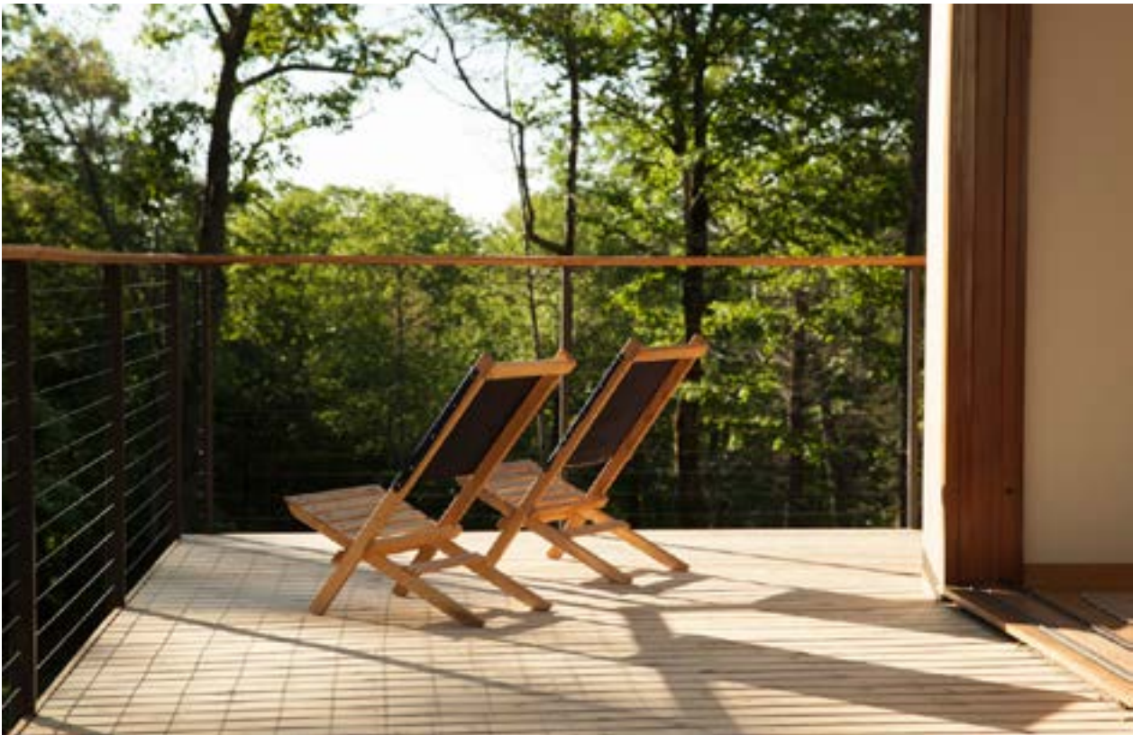
It was important that the railings at Hudson Woods be elegant but quiet. We did not want them to obscure any of the spectacular forest and mountain views. We decided to construct them using a post-and-cable system, keeping sitelines minimally interrupted. The successful assembly and detailing of the powder-coated steel posts we left in the expert hands of collaborator Andrew Becker.
